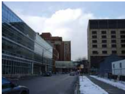
Figure 6. The Outpatient Care Centre (left) is connected to the UIC Hospital (right)
